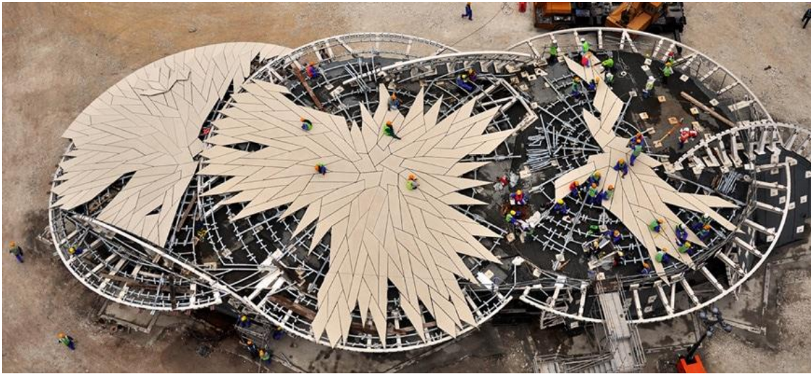
Figure 5-19: The “disks” of the museum consist of a steel frame clad with prefabricated UHPFRC panels.
