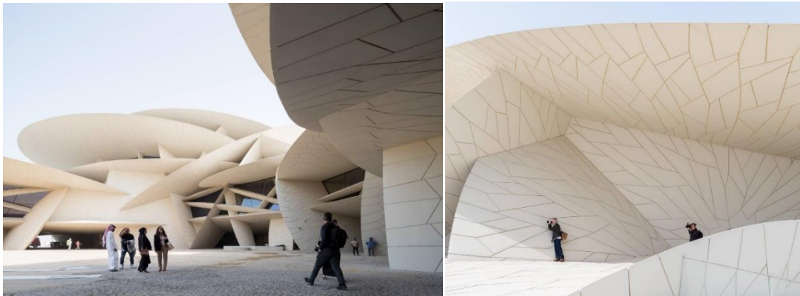
Figure 5-18: High-performance glass fiber-reinforced concrete. Source: (URL 4).
