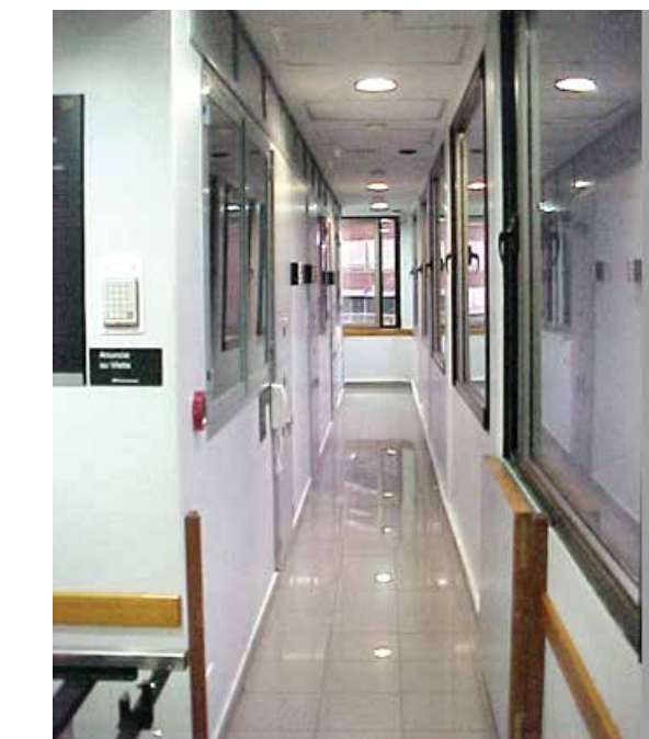
FIGURE 8. Burn Unit Peripheral Corridor With Windows Facing the Patients' Rooms
